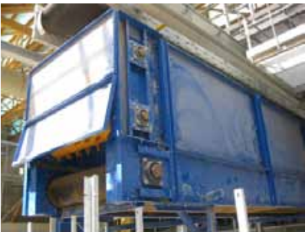
Dosing reels by the discharge side
